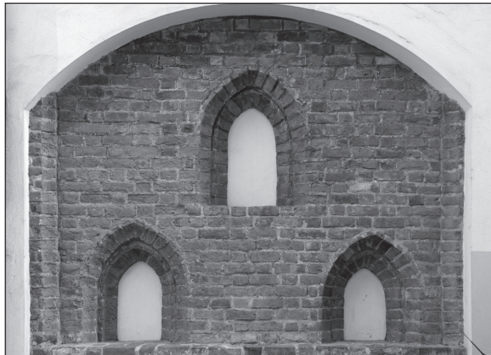
Fig. 28 Zelný trh 7, ground floor wall from format II.2 high bricks (photo archive Archaia Brno o. p. s. – inv. no. 01926-2011).
