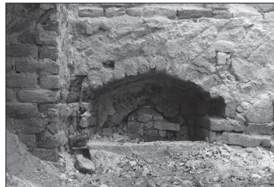
Fig. 10 Former Carthusian monastery in Královo Pole. Brick entrance from the corridor of the large cloister into the area of one of the monks' gardens from category II.2 high bricks (photo archive Archaia Brno o. p. s. – inv. no. 12555-2006).
