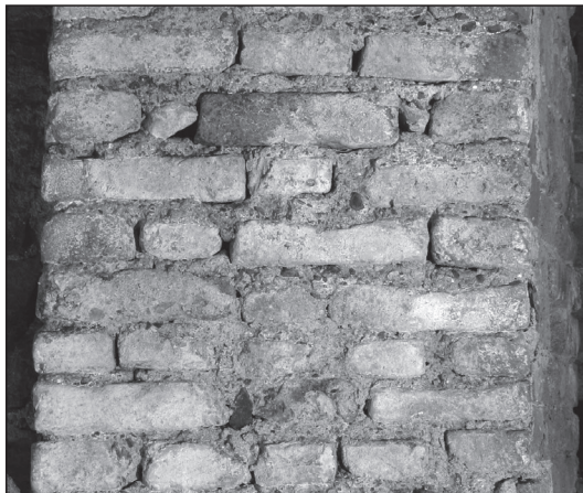
Fig. 36 Minoritská 2, surface finish of masonry wall from format I.2 bricks (photo archive Archaia Brno o. p. s. – inv. no. 2794-2004).
