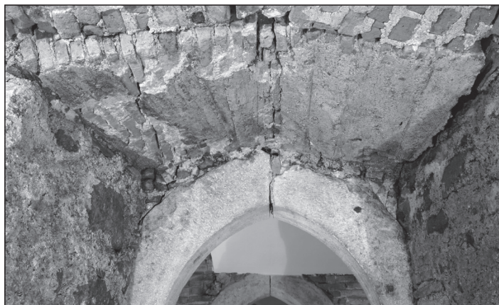
Fig. 20 Minoritská 2, discharging arch of the Gothic entrance of the basement built from format I.2 bricks (photo archive Archaia Brno o. p. s. – inv. no. 2811-2004).
