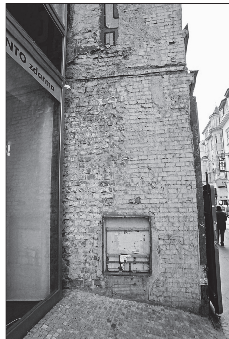
Fig. 25 Česká 10, northern perimeter wall on the ground floor built from format II.2 high bricks (photo archive Archaia Brno o. p. s. – inv. no. 118-03-23).
