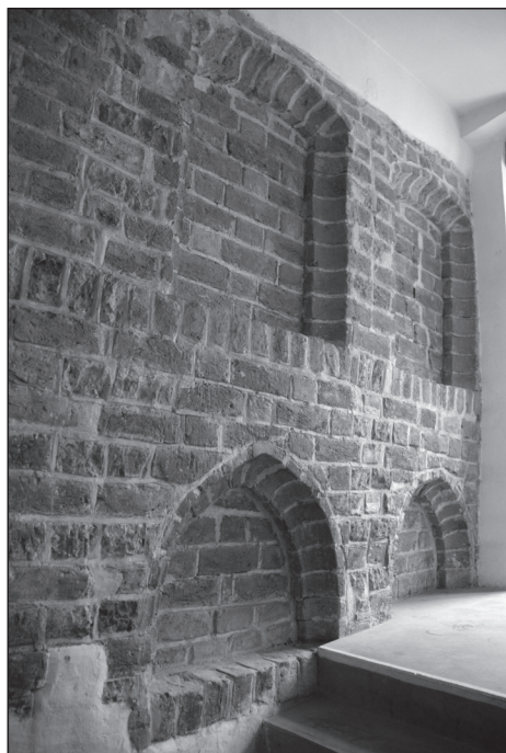
Fig. 24 The Old Town Hall, walled-up blind windows on the floor of the house from format II.2 high bricks (photo archive Archaia Brno o. p. s. – inv. no. 06982-2012).
