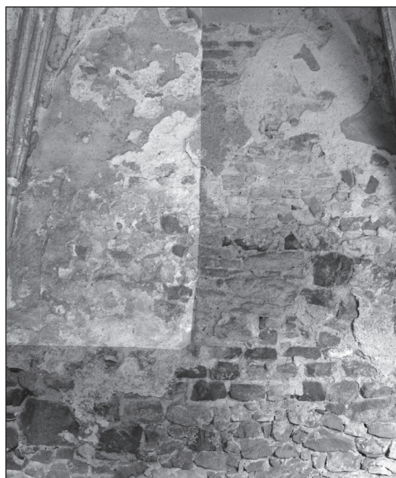
Fig. 47 Dolní Kounice, former Church of the Virgin Mary of the "Rosa Coeli" convent of Cistercian nuns. Western perimeter wall of the cruciform corridor – masonry lining of the Gothic window (photo archive Archaia Brno o. p. s. – inv. no. 25363-2017).
