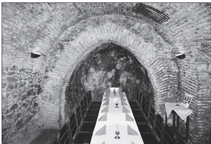
Fig. 17 Petrov 2, arch in the basement built from format I.2 bricks (photo archive Archaia Brno o. p. s. – inv. no. 113-01-24).
