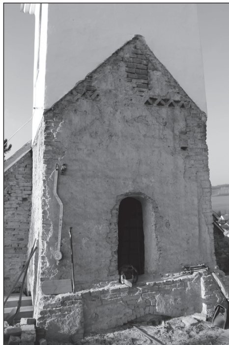
Fig. 41 Staré Hvězdlice, All Saints' Church, tower after removal of the later truss (photo archive Archaia Brno o. p. s. – inv. no. 23303-2009).
