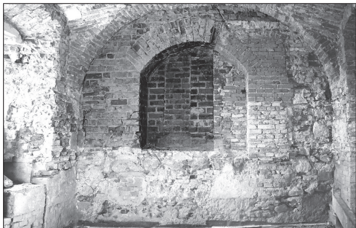
Fig. 26 Petrov 3, basement arch built from Gothic format II.2 high bricks (photo archive Archaia Brno o. p. s. – inv. no. 054-02-020).
