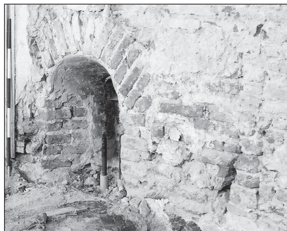
Fig. 5 Minorite convent, brick arch of a Roman window from format I.2 bricks (photo archive Archaia Brno o. p. s. – inv. no. A04-98-041).
