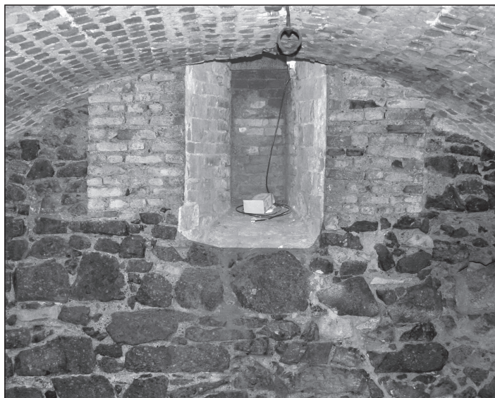
Fig. 21 Minoritská 2, candle niche in the basement from format I.2 bricks (photo archive Archaia Brno o. p. s. – inv. no. 3226-2004).
