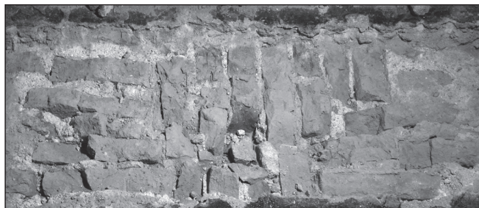
Fig. 13 The Old Town Hall, crown of the vault of the so-called treasure chamber built from format I.2 bricks (photo archive Archaia Brno o. p. s.)
