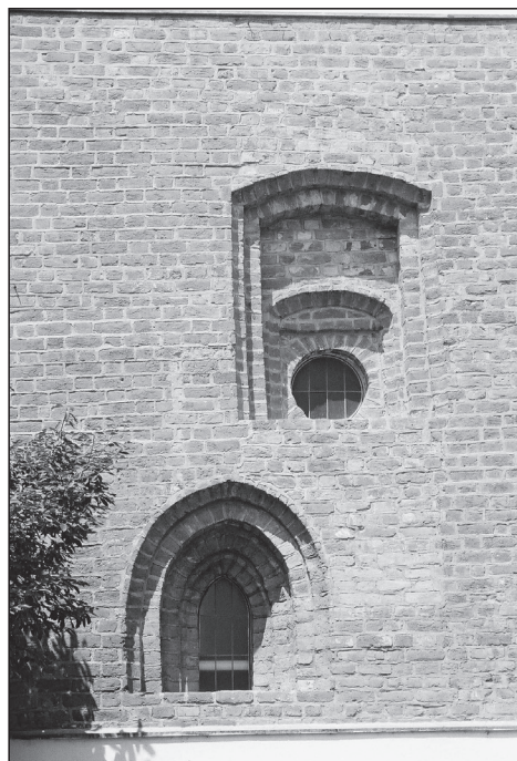
Fig. 23 The Old Town Hall, brick walls on the floor of the house from format II.2 high bricks (photo archive Archaia Brno o. p. s. – inv. no. 175-02-019).
