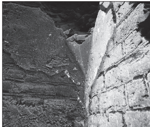
Fig. 38 St Thomas' Church, original pointing of the inner corner of a buttress at the southern wall built from format II.1 bricks (photo archive Archaia Brno o. p. s. – inv. no. 06083-2014).
