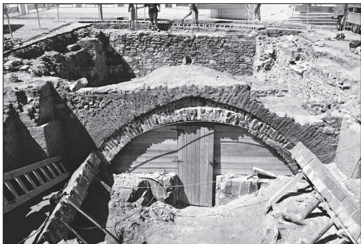
Fig. 16 Dominikánské náměstí 2 (house of the Cistercian nuns from Staré Brno), arch bearing the ground floor partition built from format I.3 low bricks (photo archive Archaia Brno o. p. s. – inv. no. 059-01-028).
