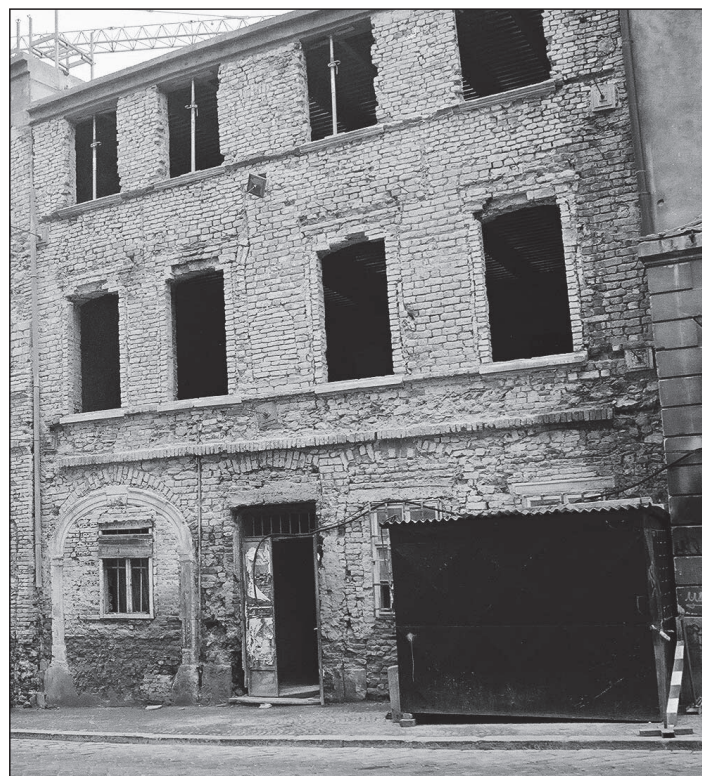
Fig. 29 Dominikánská 7, front up to the floor level built from format II.2 high bricks. A brick arch preserved above the portal from the Classicist period (photo archive Archaia Brno o. p. s. – inv. no. A00-10-310).
