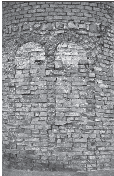
Fig. 40 Staré Hvězdlice, All Saints' Church, presbytery with plaster strips from hewn bricks (photo archive Archaia Brno o. p. s. – inv. no. 1077-2009).
