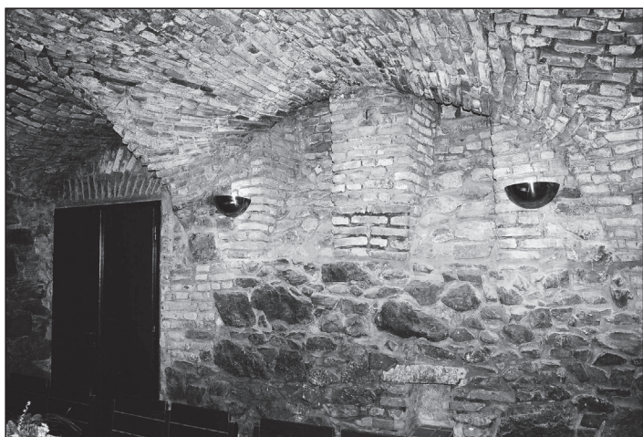
Fig. 18 Petrov 2, lining of the small windows on the eastern side of the basement from format I.2 bricks (photo archive Archaia Brno o. p. s. – inv. no. 120-01-20).
