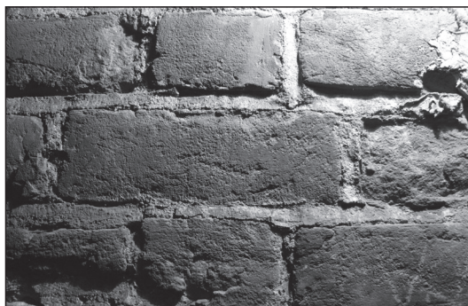
Fig. 37 Staré Brno – Church of the Assumption, original pointing of the masonry wall from format II.1 bricks preserved in the roof truss area (photo archive Archaia Brno o. p. s. – inv. no. 07040-2016).
