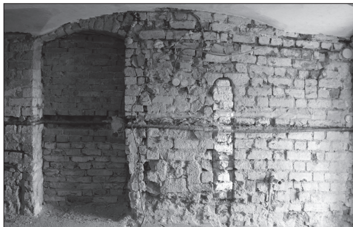
Fig. 27 Petrov 3, exterior side of the wall from Gothic format II.2 high bricks (photo archive Archaia Brno o. p. s.).
