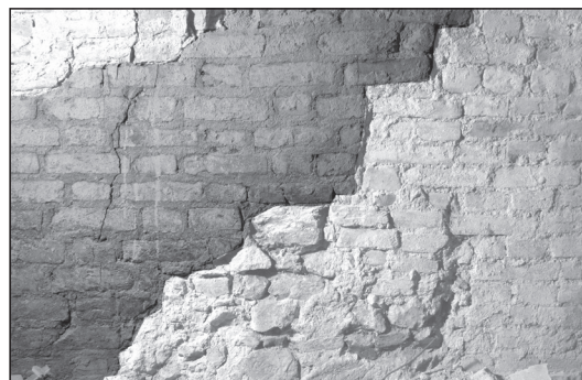
Fig. 39 Orlí 16, surface finish of masonry wall on the floor – format II.2 bricks (photo archive Archaia Brno o. p. s. – inv. no. 04496-2006).
