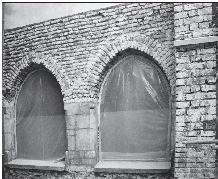
Fig. 4 Former Dominican monastery, brick arcades of the southern wing of the cloister corridor from format I.2 bricks (photo archive Archaia Brno o. p. s. – inv. no. 027-02-022).
