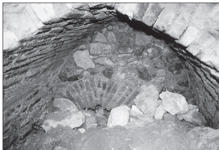
Fig. 15 Kapucinské náměstí – cellar with vault from Gothic format I.2 low bricks (photo archive Archaia Brno o. p. s. – inv. no. 021-06-12).
