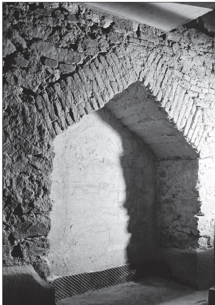
Fig. 19 Dominikánská 9, discharging arch of the basement built from format I.2 bricks (photo archive Archaia Brno o. p. s. – inv. no. 109-01-018).
