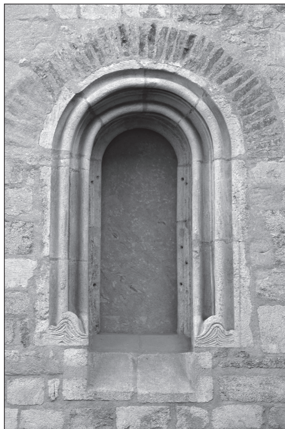
Fig. 3 Brno-Zábrdovice, Chapel of St. Kunigunde. Segmented arch above the chapel window from category I low bricks (photo archive Archaia Brno o. p. s. – inv. no. 01093-2014).
